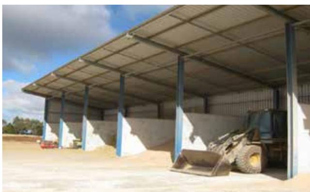
**Figure 88.** Design individual bays to cater for typical delivery truck volumes – store feed undercover
