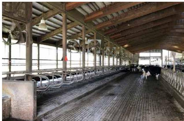
**Note:** the high open side walls and fans located over the resting area.
