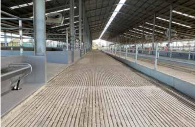
**Note:** Grooves cut into the concrete in the direction of the alley.
