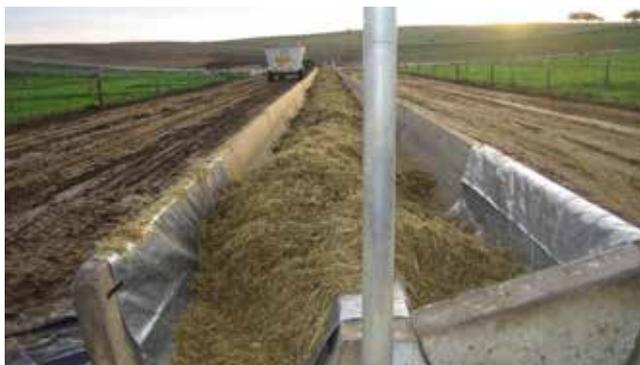
*Formed earthen feedpad with concrete troughs*
