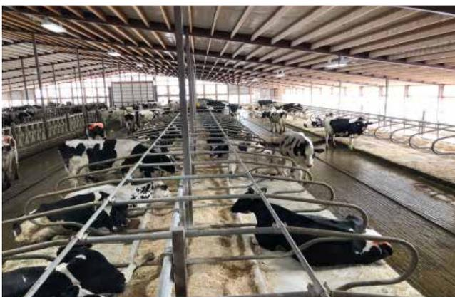
Note the double head-to-head row of stalls adjacent to the feed alley.
