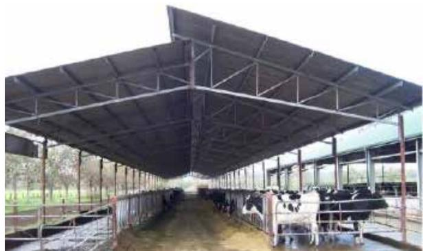
Concreted overlapping roofed feedpad
