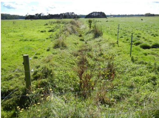
Trench drains should be fenced from stock and machinery. They should be sprayed out in spring and autumn and cleared out with machinery when clogged with growth or silt. If not maintained, drains stop working (*left*).
