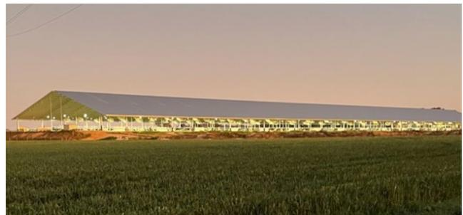
Lights are fitted down the centre of the shed. They turn on at 2:30am to wake up the three-times group of cows prior to milking at 3:15am and switch off again at sunrise when the light intensity in the shed rises above 150 lux. If the light intensity in the shed falls below 200 lux at any time during the day, the lights will turn on. In the evening the lights turn on at about 6:30pm and stay on until 10:00pm.
