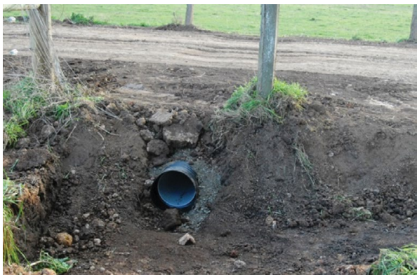
These photos illustrate construction of a culvert to drain water under laneway (Copyright Jakob Malmo)
