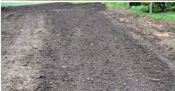
In this example pulverised wood and sawdust create transition zone drainage
