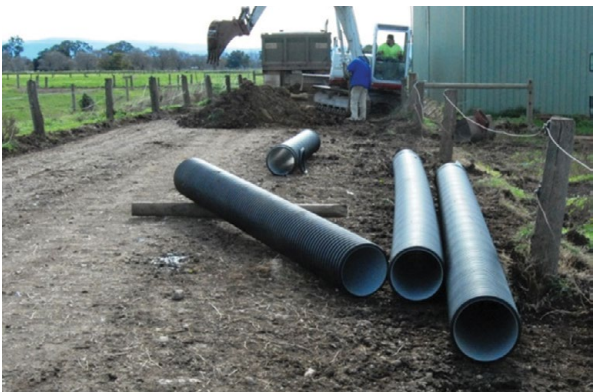
These photos illustrate construction of a culvert to drain water under laneway (Copyright Jakob Malmo)
