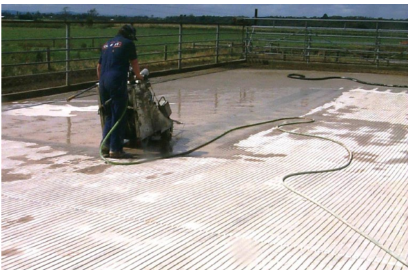
Grooving the yard in the direction of cow flow
