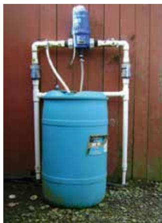
Figure 23. Dosatron™ in-line dispenser
