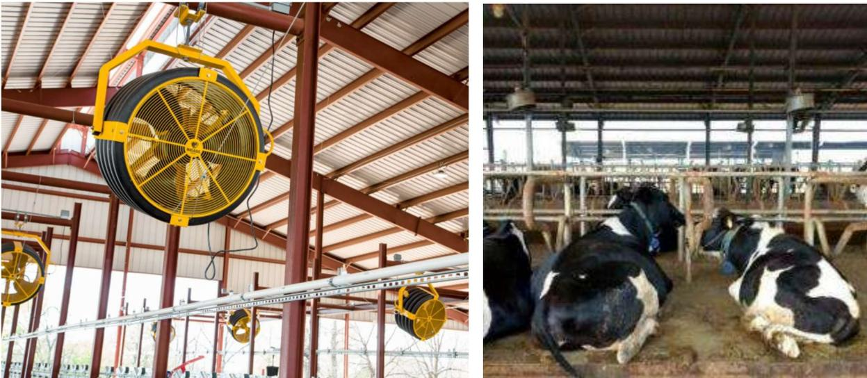
Figure 22. Oscillating box fans directing air down onto cows and bedding area. Source (Left Ref 12. Right P Chamberlain, India)
