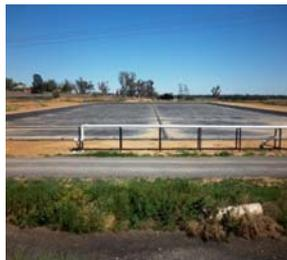
A 14ML covered anaerobic lagoon at Bungowanah. A 6,000 sow "breeder only" piggery 2012
