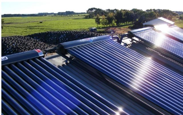
Image Example of evacuated tube hot water system on a dairy farm.
