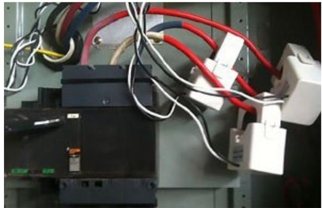
Figure 2 Unit to log and record energy use
