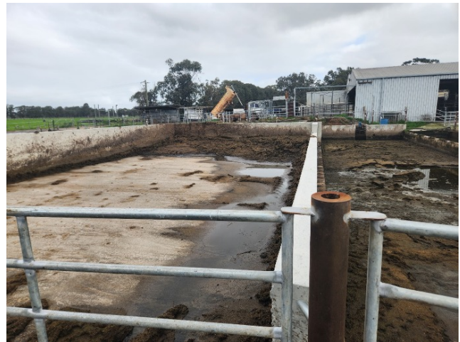
Effluent Solids Storage Pad Evans Dairy Busselton.
